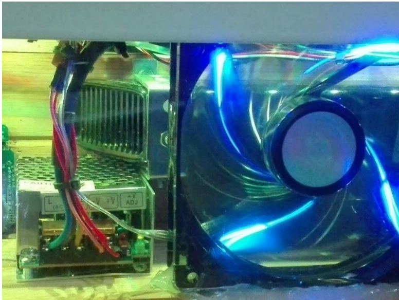
Figure B.5: Interior Fan
